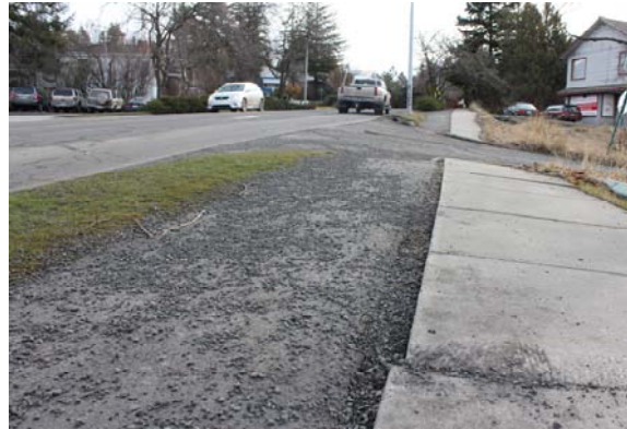
Deep Construction Joints on the Stadium Way path may pose a risk to bicyclists.
